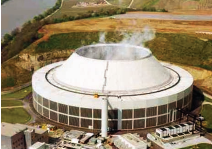
Wet-Dry Hybrid Cooling —The wet-dry hybrid cooling tower offers efficient cold water temperatures with reduced visible plume and enhanced water conservation.
